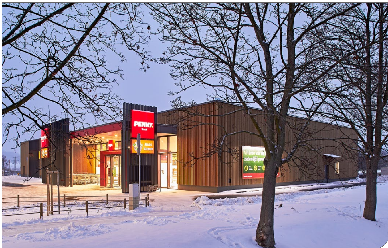
Figure 83. ThermoWood® products at Supermarket in Skuteč, CZ.
