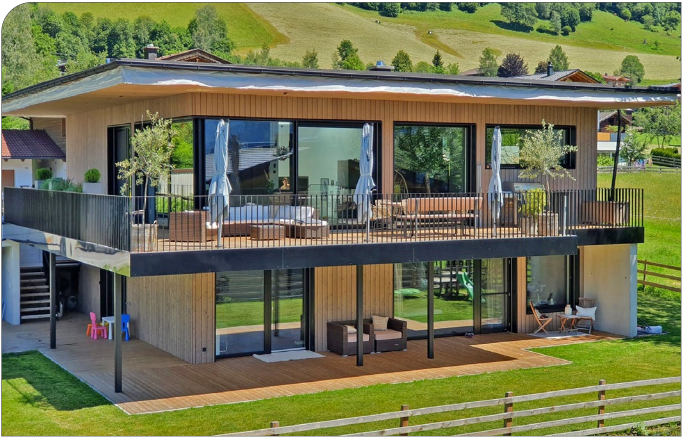
Figure 75. ThermoWood® exterior cladding in Austria.
