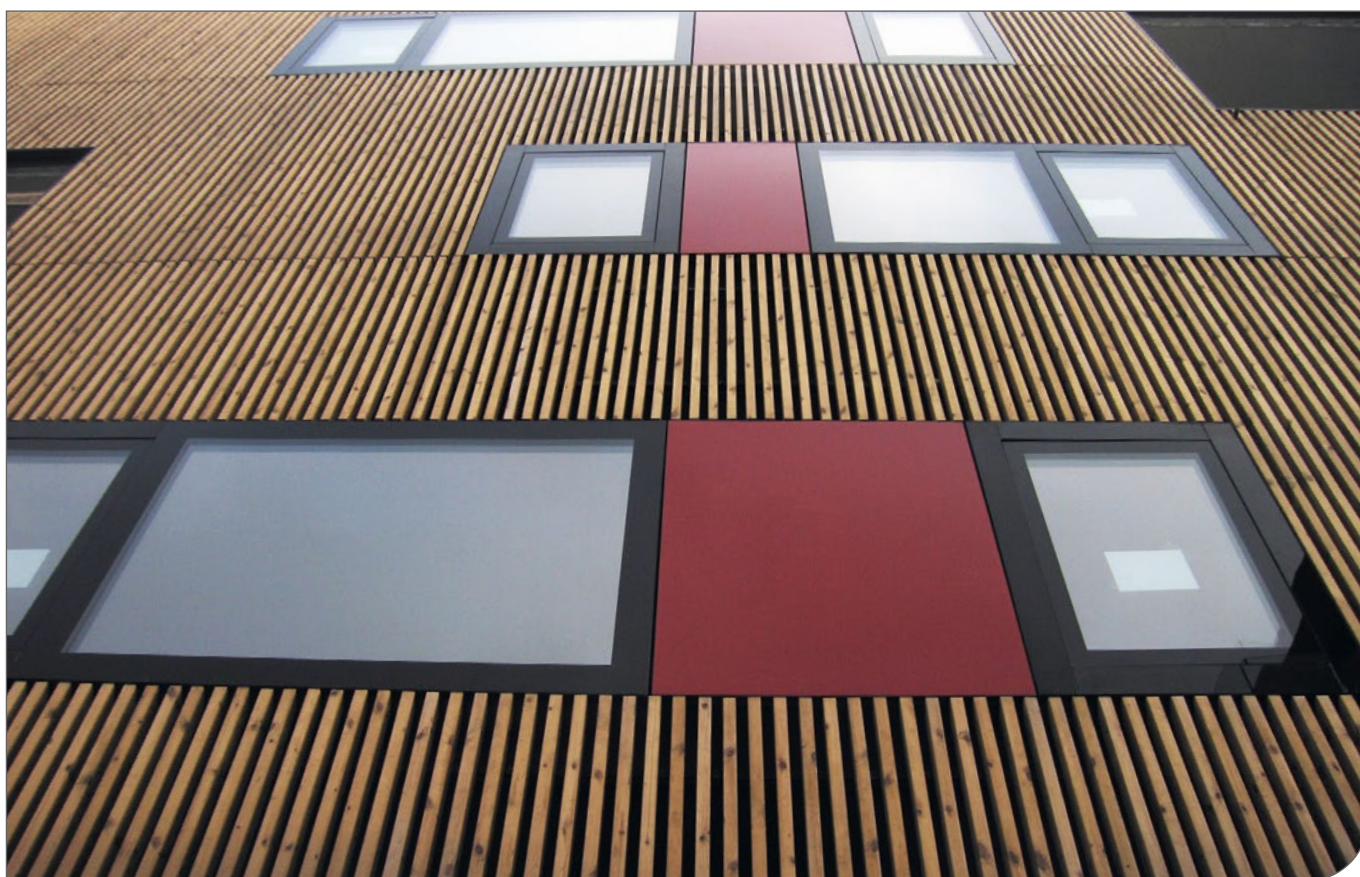
Figure 63. Exterior cladding made of ThermoWood® products.
