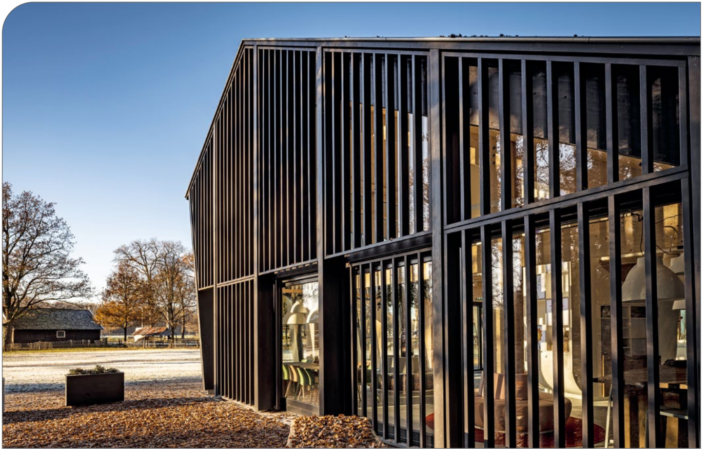
Figure 69. ThermoWood® exterior cladding (Netherlands).
