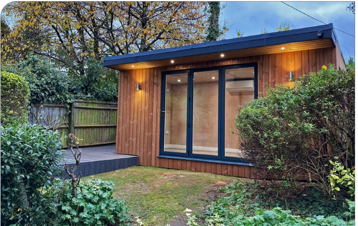
Figure 76. ThermoWood® exterior cladding in the UK.
