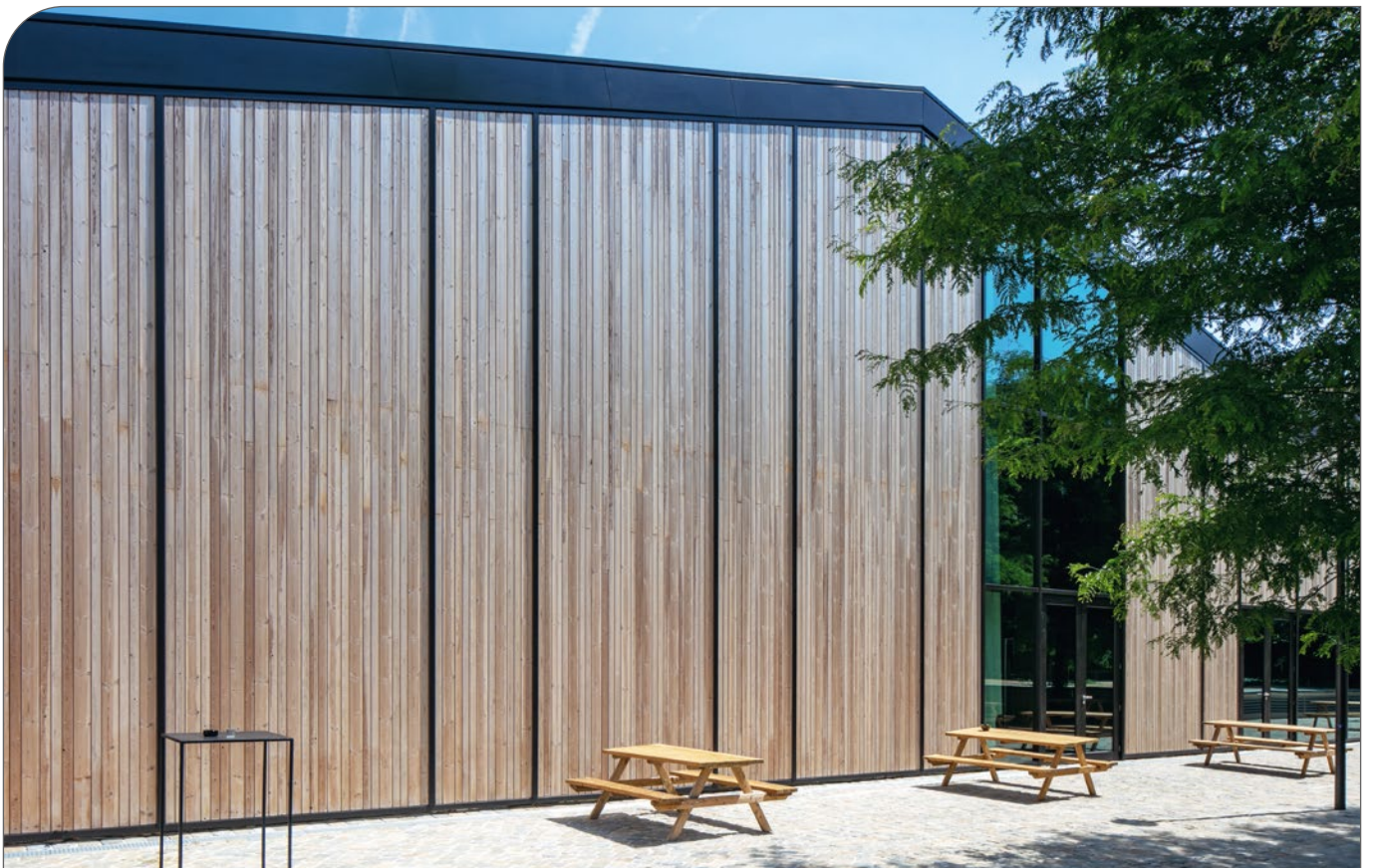
Figure 70. ThermoWood® exterior cladding (Belgium).
