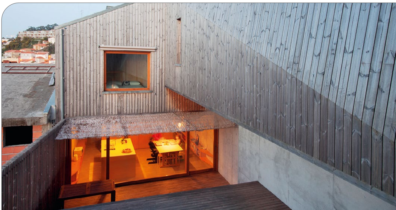
Figure 62. ThermoWood® exterior wall cladding with a naturally weathered appearance in Portugal.
