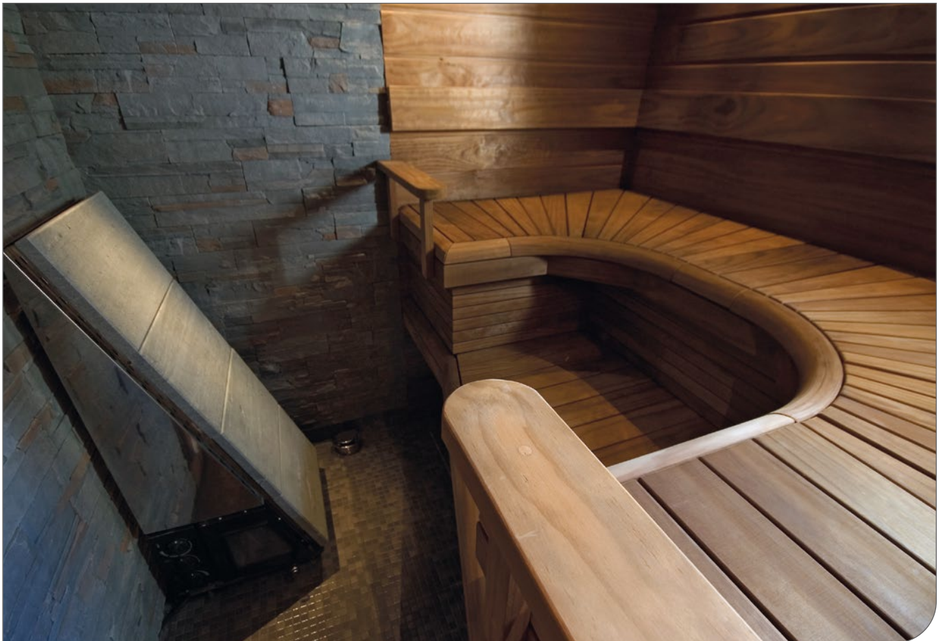
Figure 43. Sauna structures made of ThermoWood® products.
