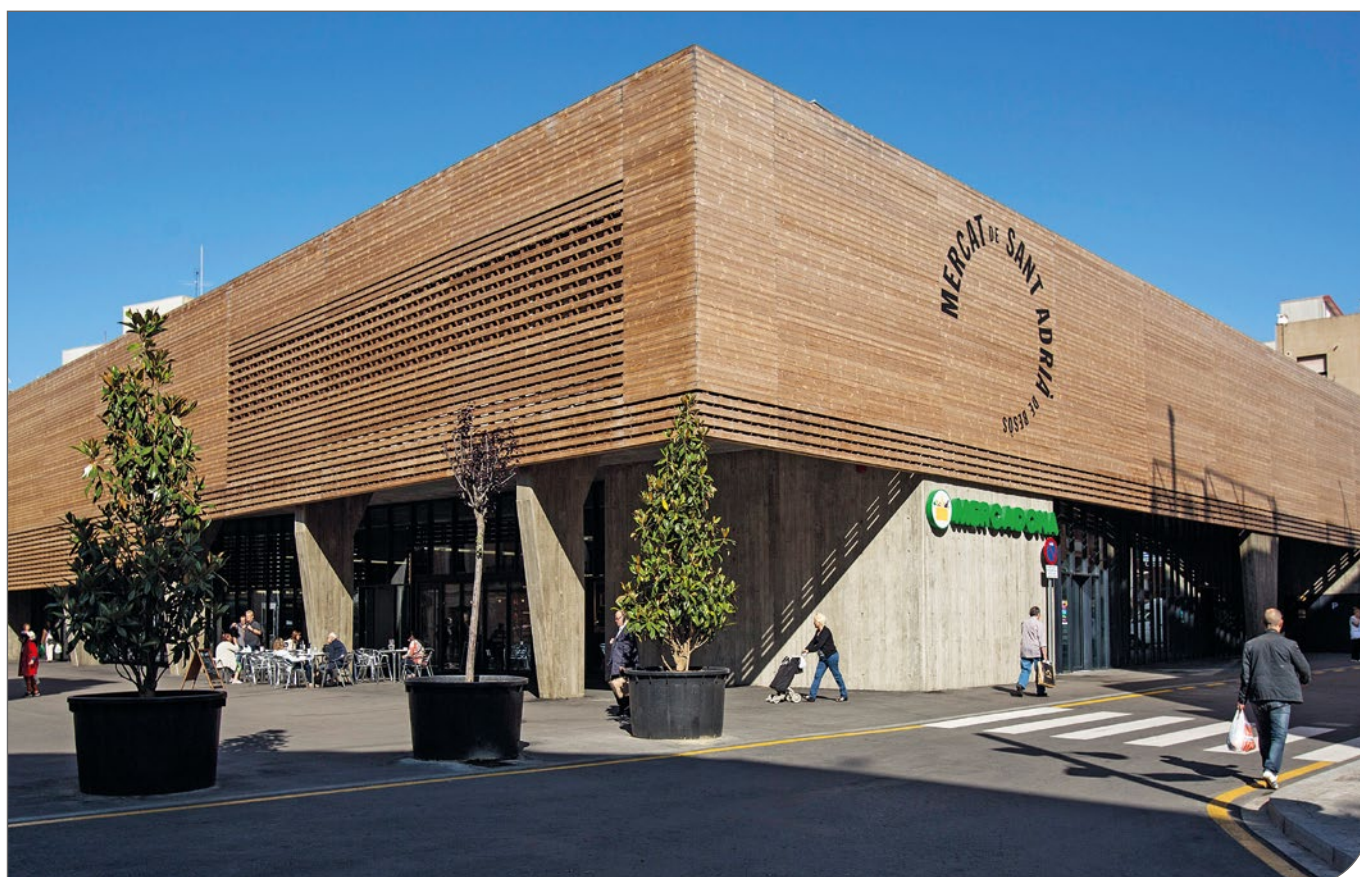
Figure 64. ThermoWood® exterior wall cladding on a Spanish shopping centre.
