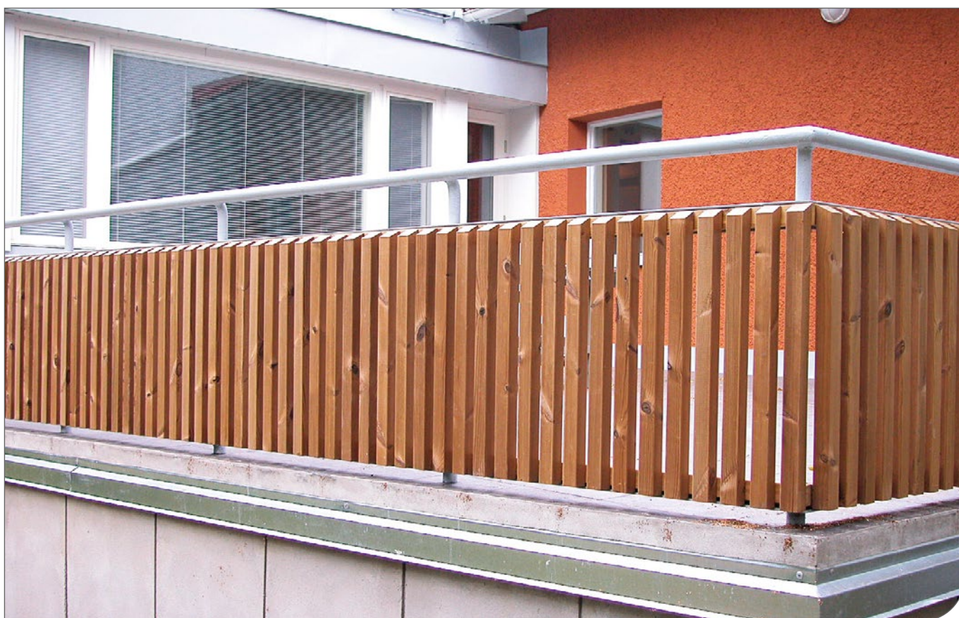
Figure 67. ThermoWood® battens on a balcony railing.
