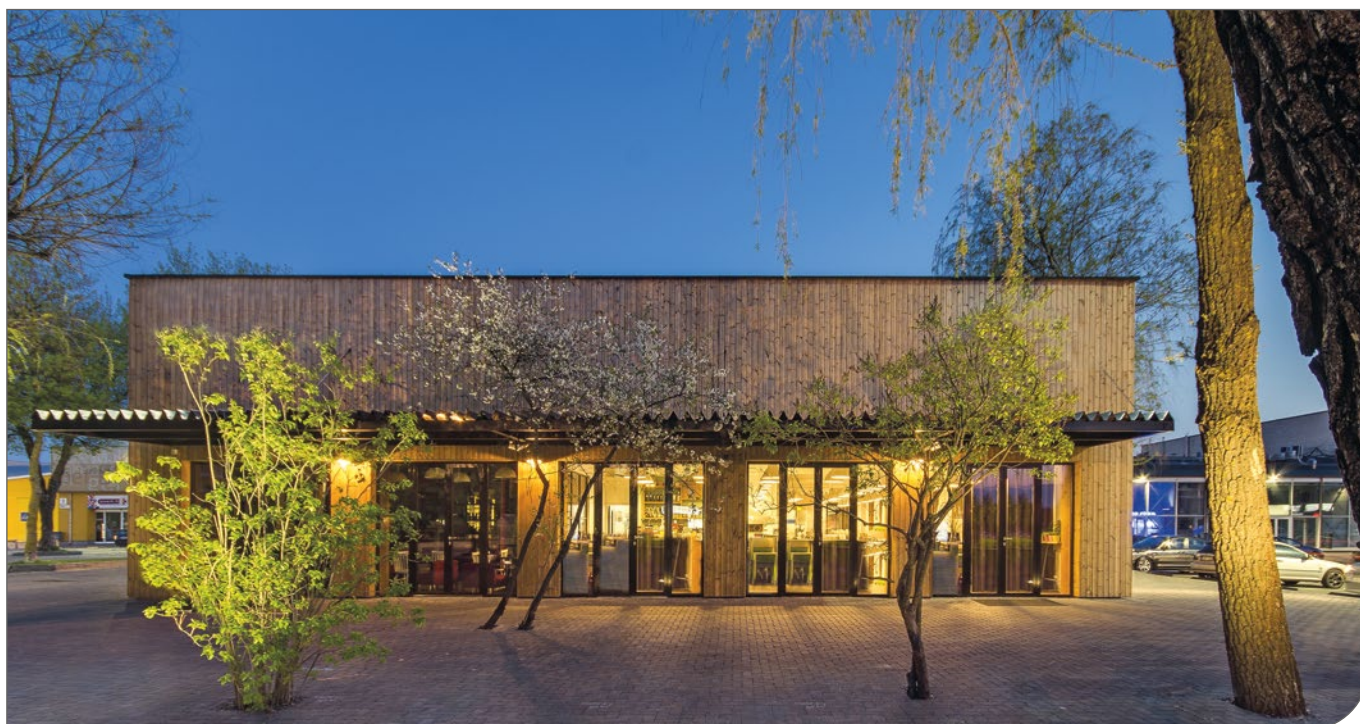
Figure 60. ThermoWood® exterior wall cladding on a Lithuanian restaurant.
