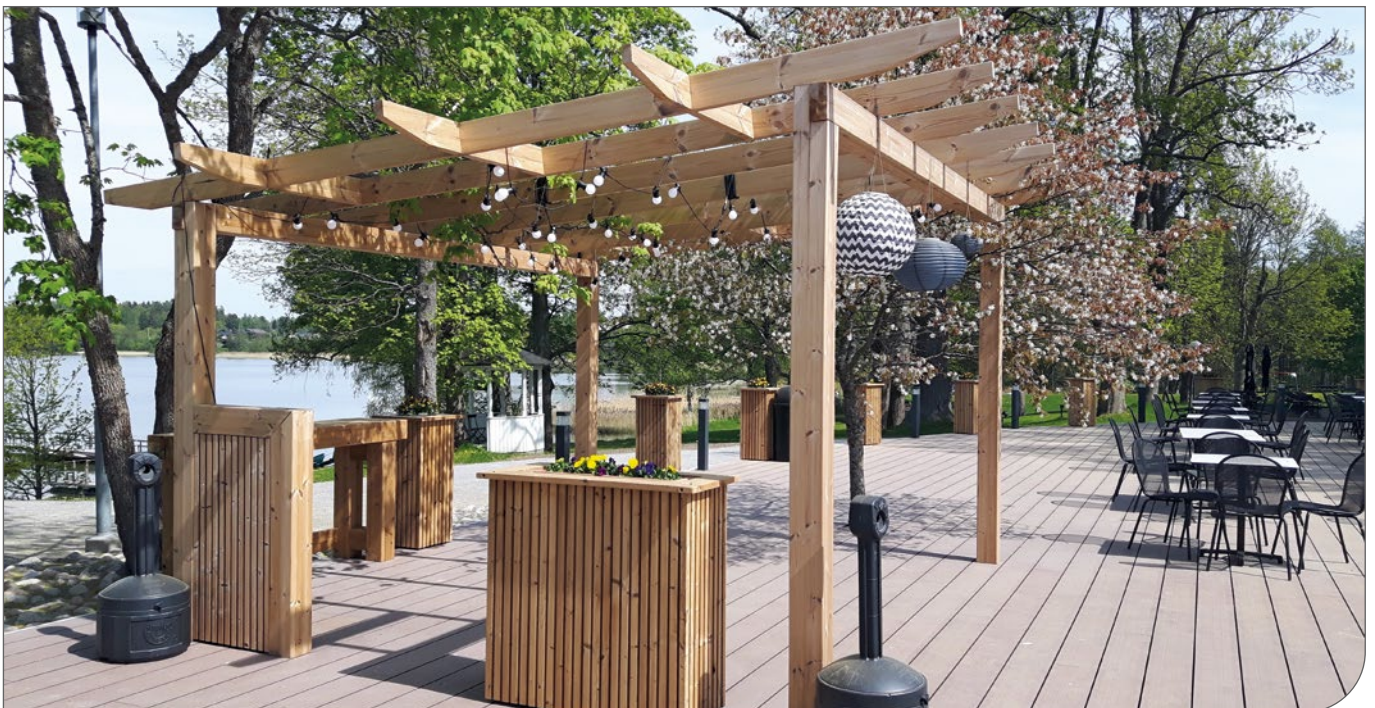
Figure 32. ThermoWood® glulam beams in pergola structure
