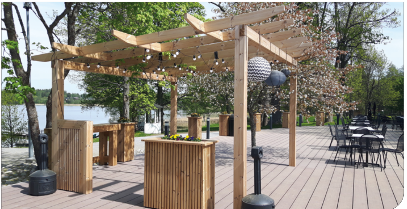
Figure 33. ThermoWood® glue beams in pergola structure
