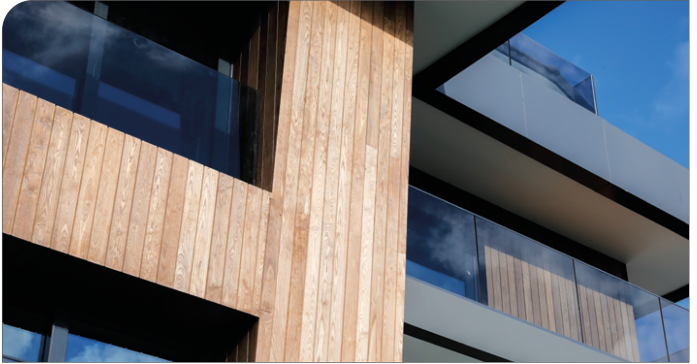
Figure 60. Exterior cladding made of ThermoWood® products. (Turkey).
